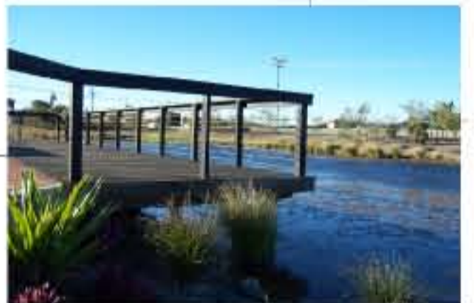
Timber Viewing Deck
